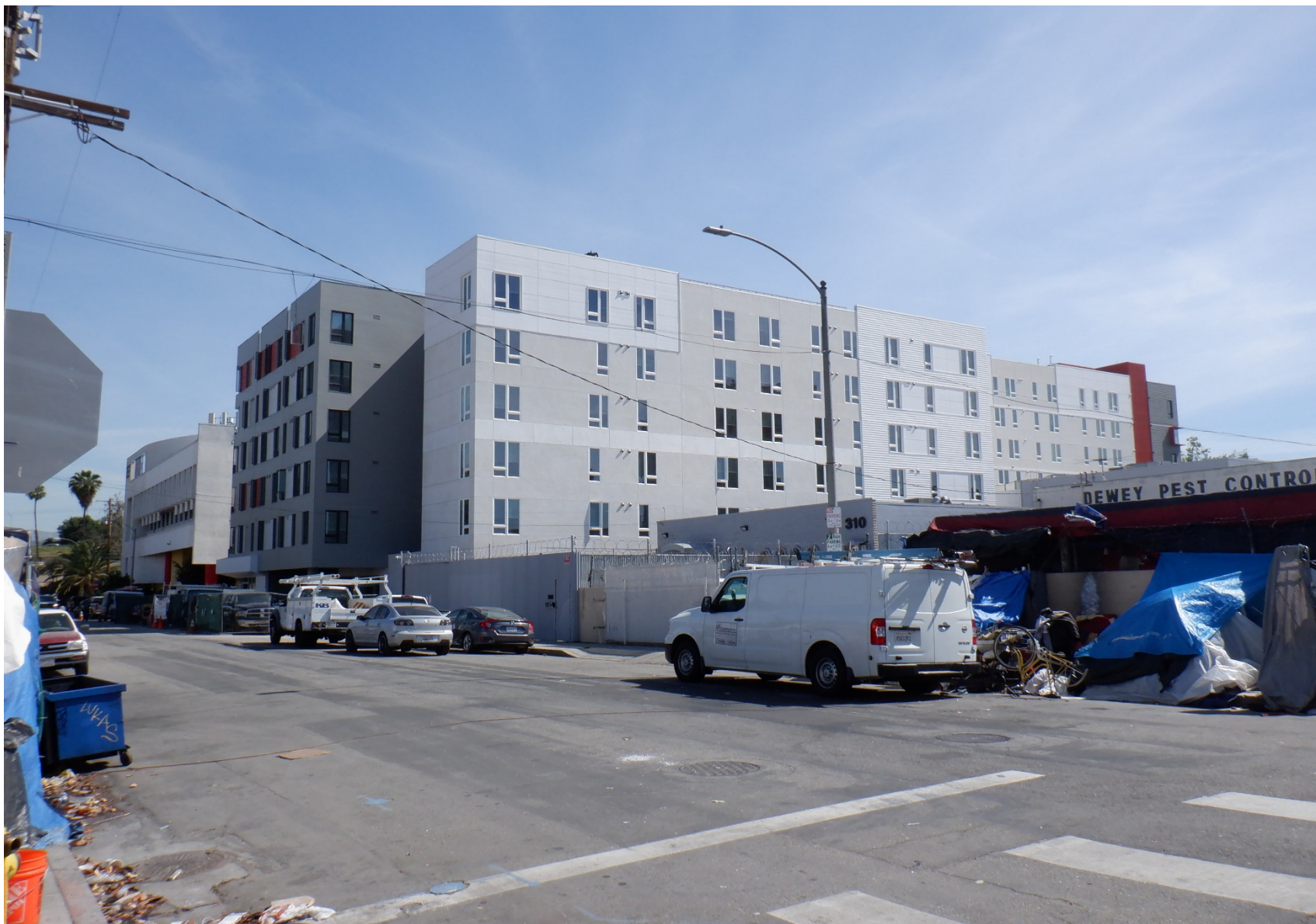
Path Metro Phase 2. View of site at corner of Beverly Blvd & Madison Ave.
