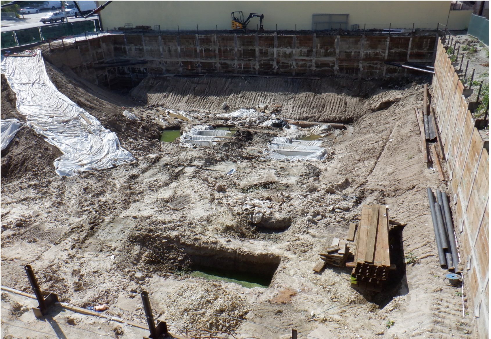
View from inside of the construction fence at 433 S Vermont.
