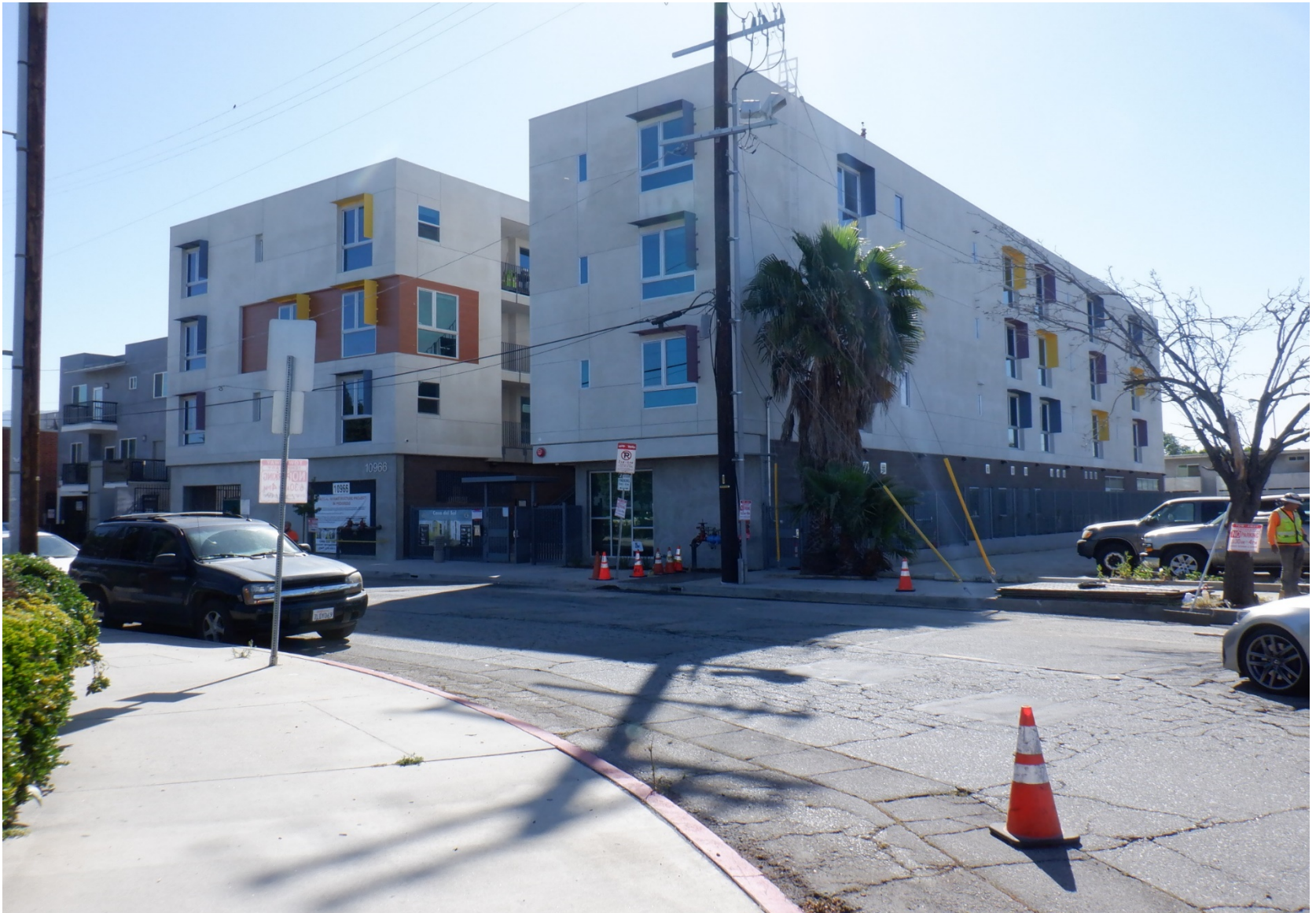
Located at 10966 Ratner St. View from across street of site.
