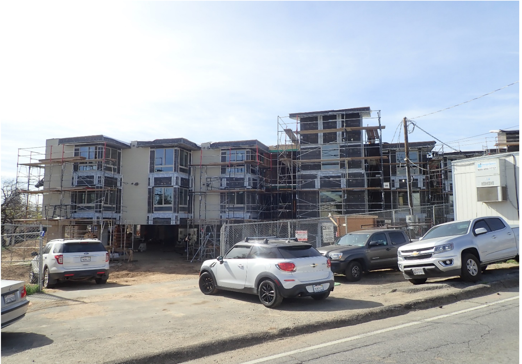
View of the two buildings from front of the site at 13574 Foothill Blvd.
