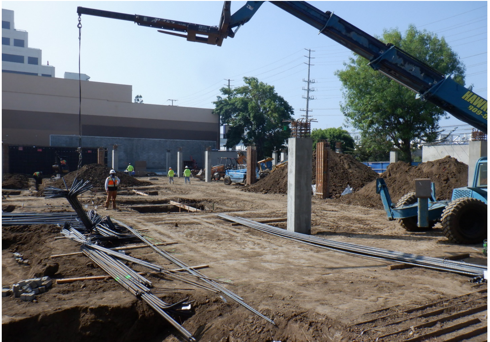
View from inside the construction fence at 11950 W. Missouri St.
