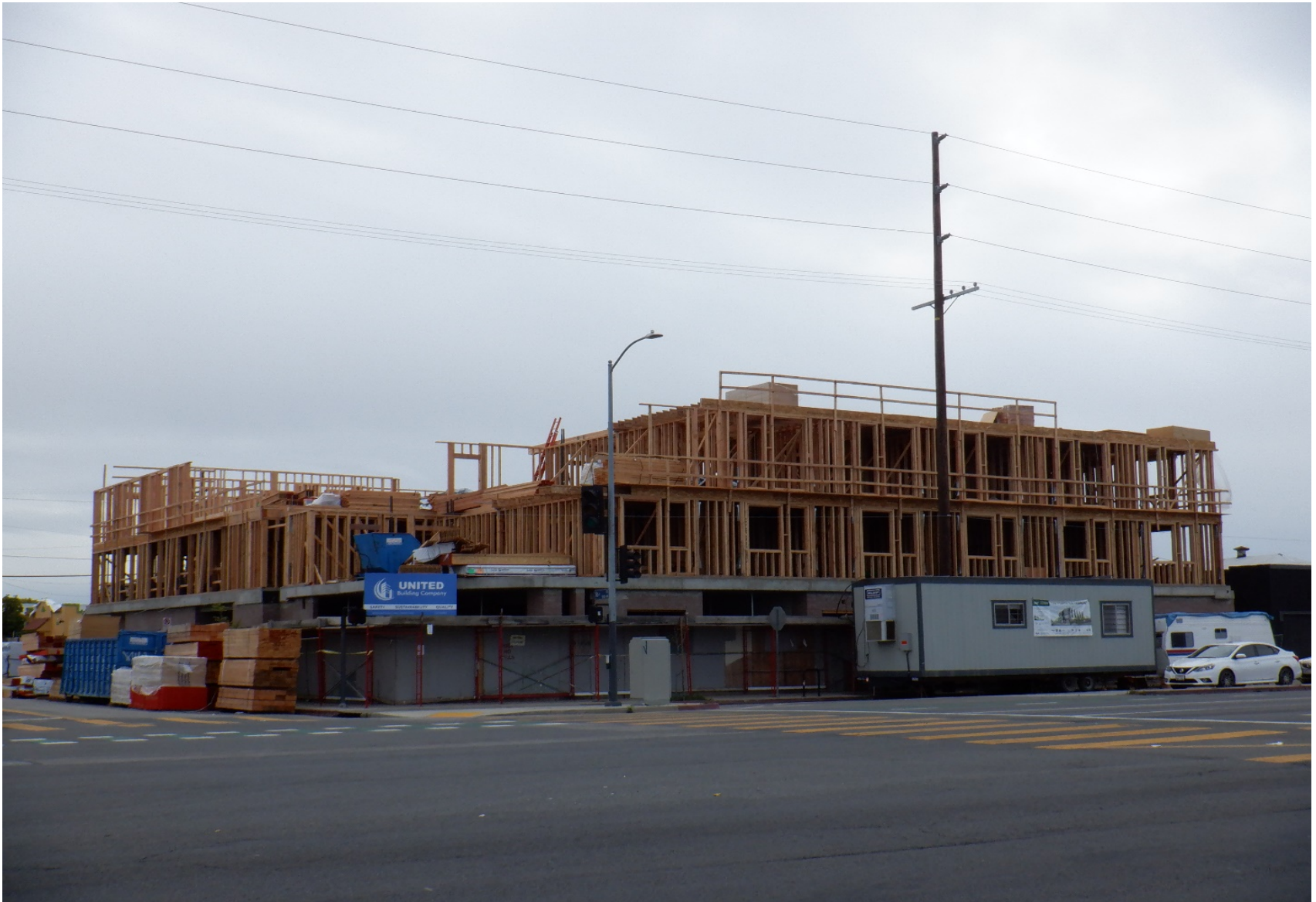
View from overhead of the construction site at 7600 S Vermont.
