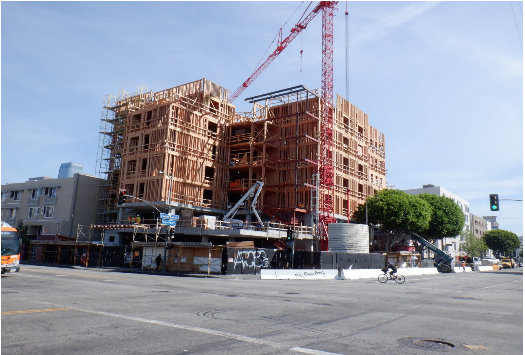
Located at 519 E 7 th St. View from inside the construction fence on 7 th St.
