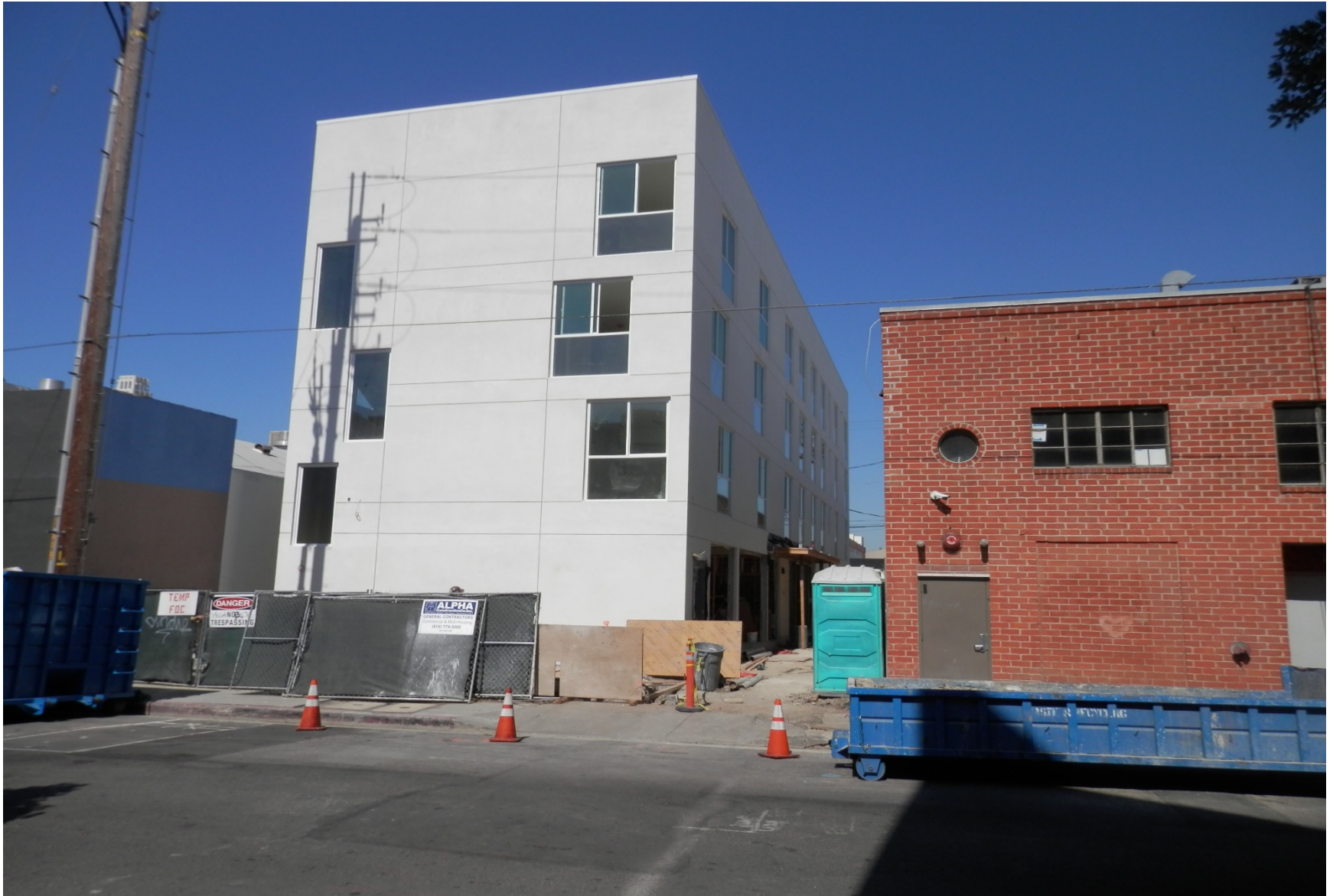
Located at 1119 N. Mc Cadden Pl. View from the front of site.
