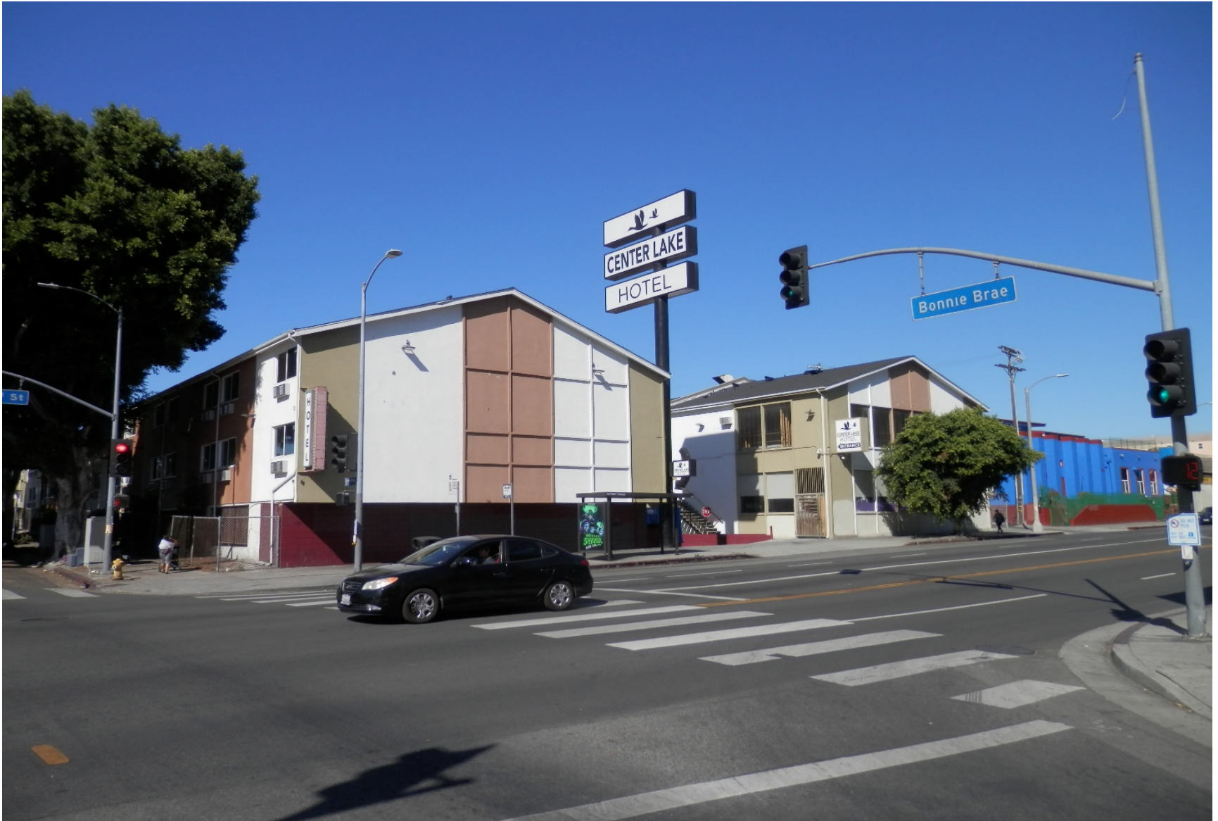
View from across the street at 1906 W 3 rd St .
