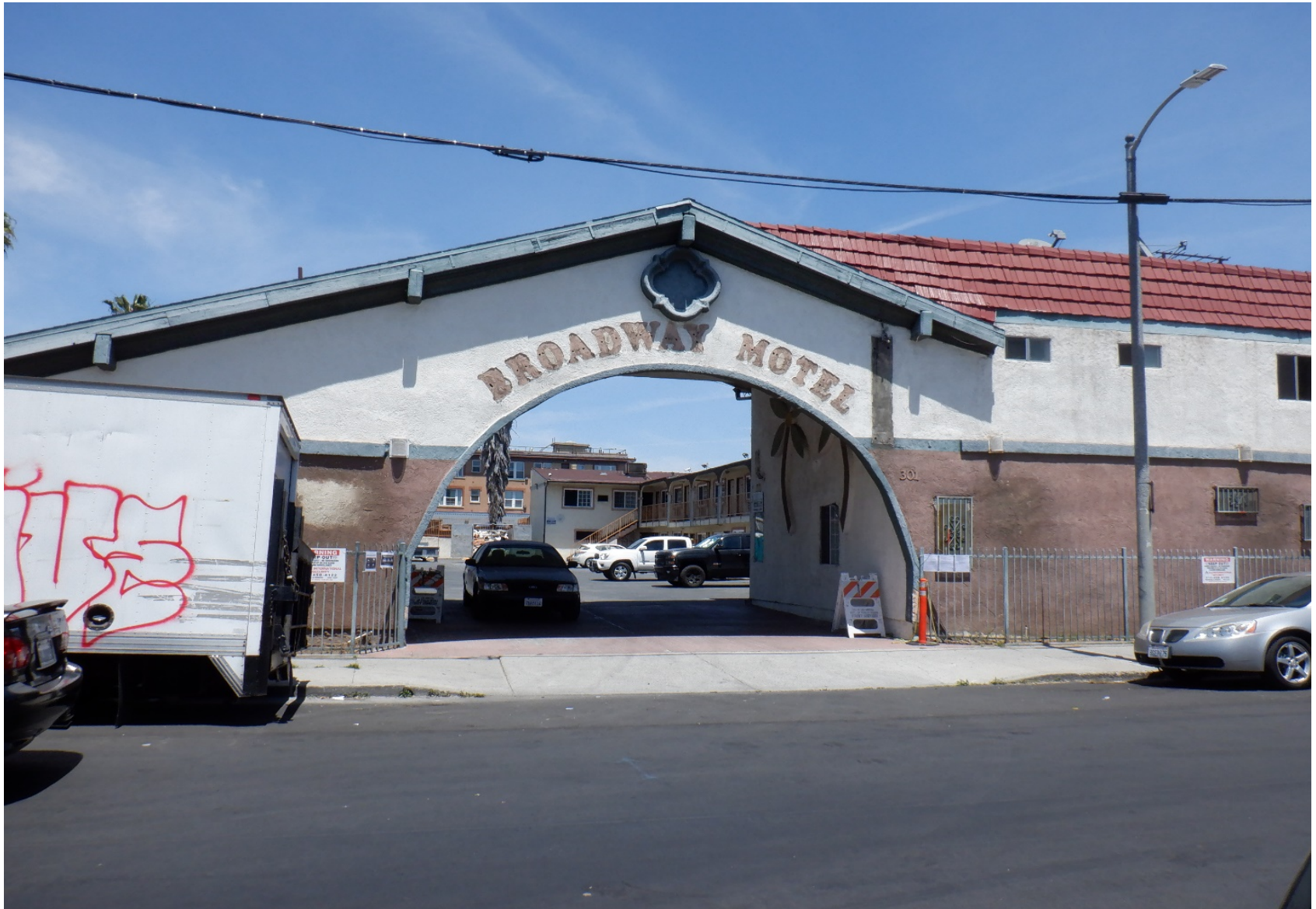
View from across the street at 301 W 49 th St .
