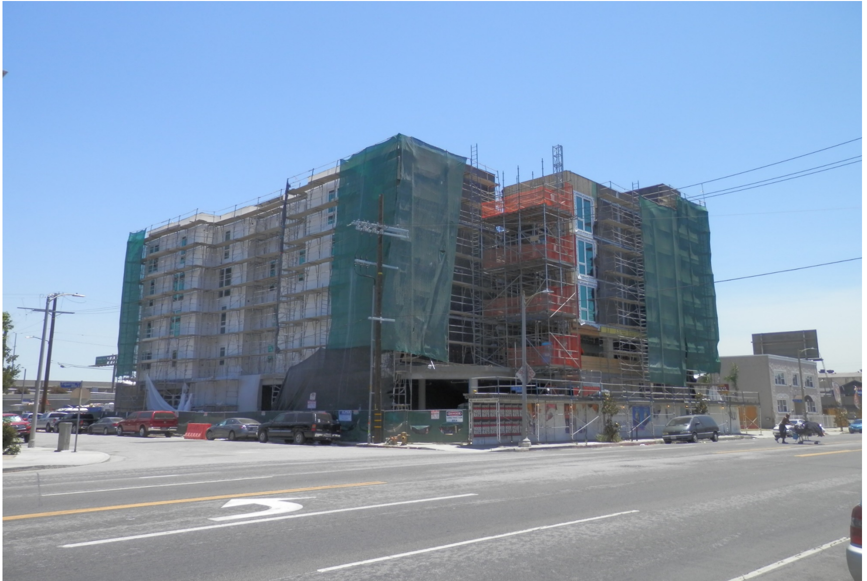
Located at 4050-60 S. Figueroa St. View from across the street of site.
