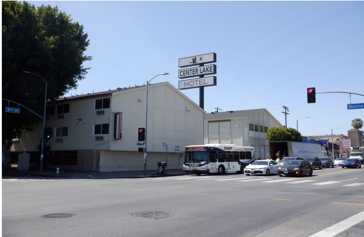
View from across the street at 1906 W 3 rd St.
