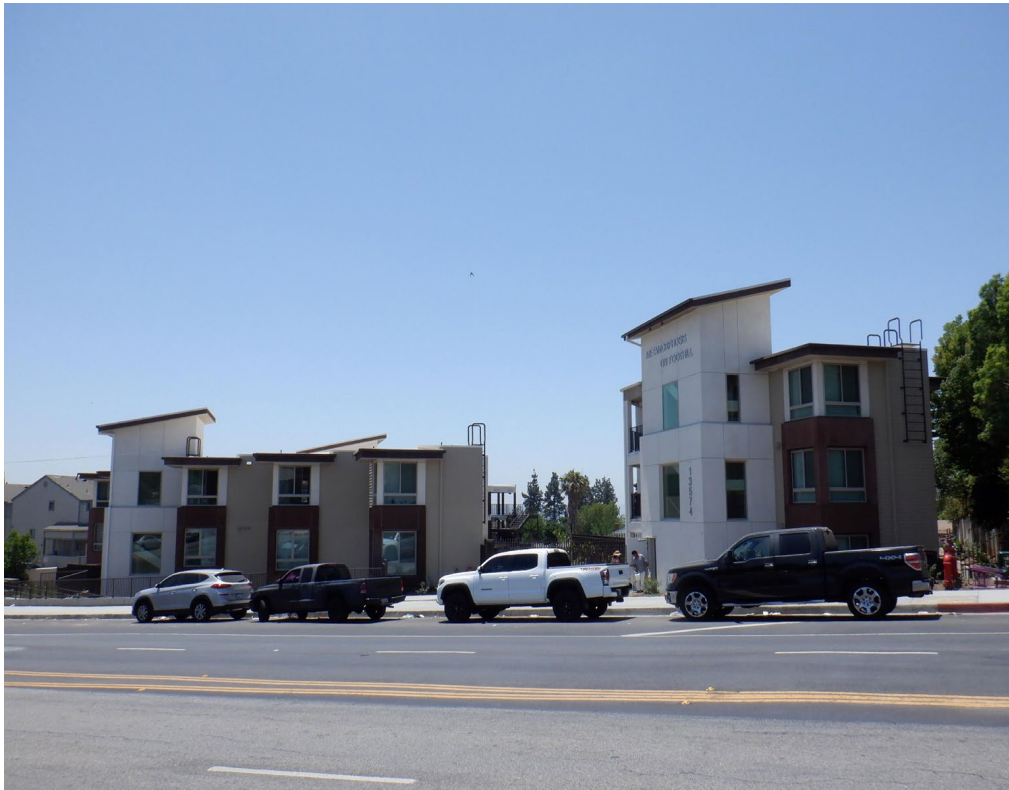
View of the buildings from the front of the site at 13574 Foothill Blvd.
