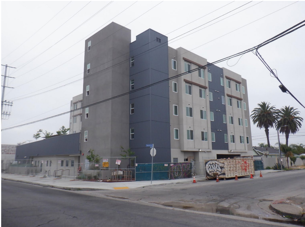
View from across the street at Florence Ave & Towne St.
