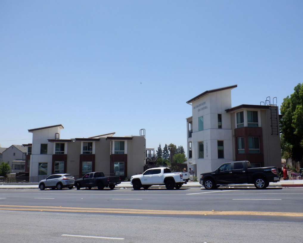
View of the buildings from the front of the site at 13574 Foothill Blvd.
