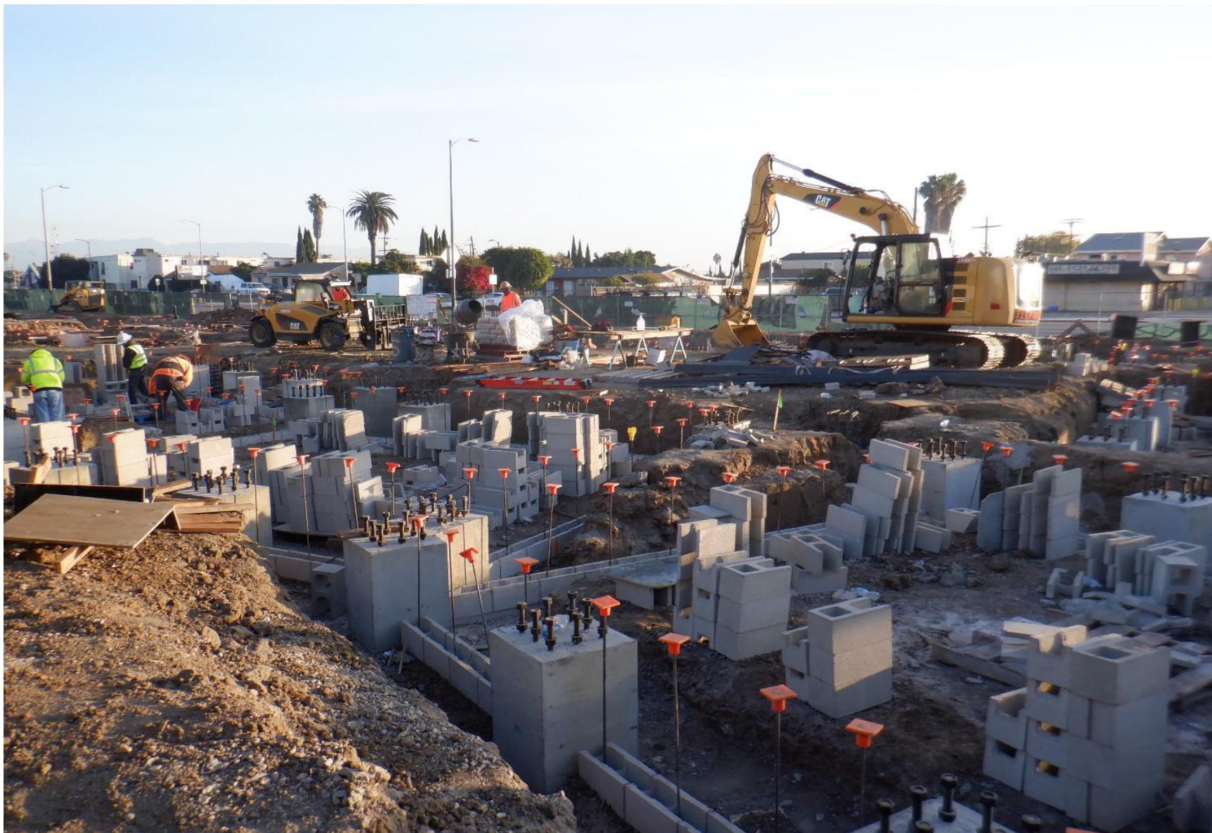
View from inside the fence at 238 W. Imperial Hwy.
