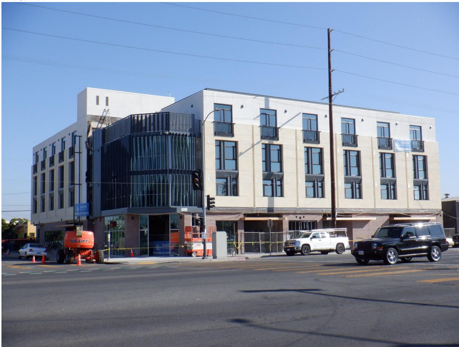
View from across the street at 7600 S Vermont.
