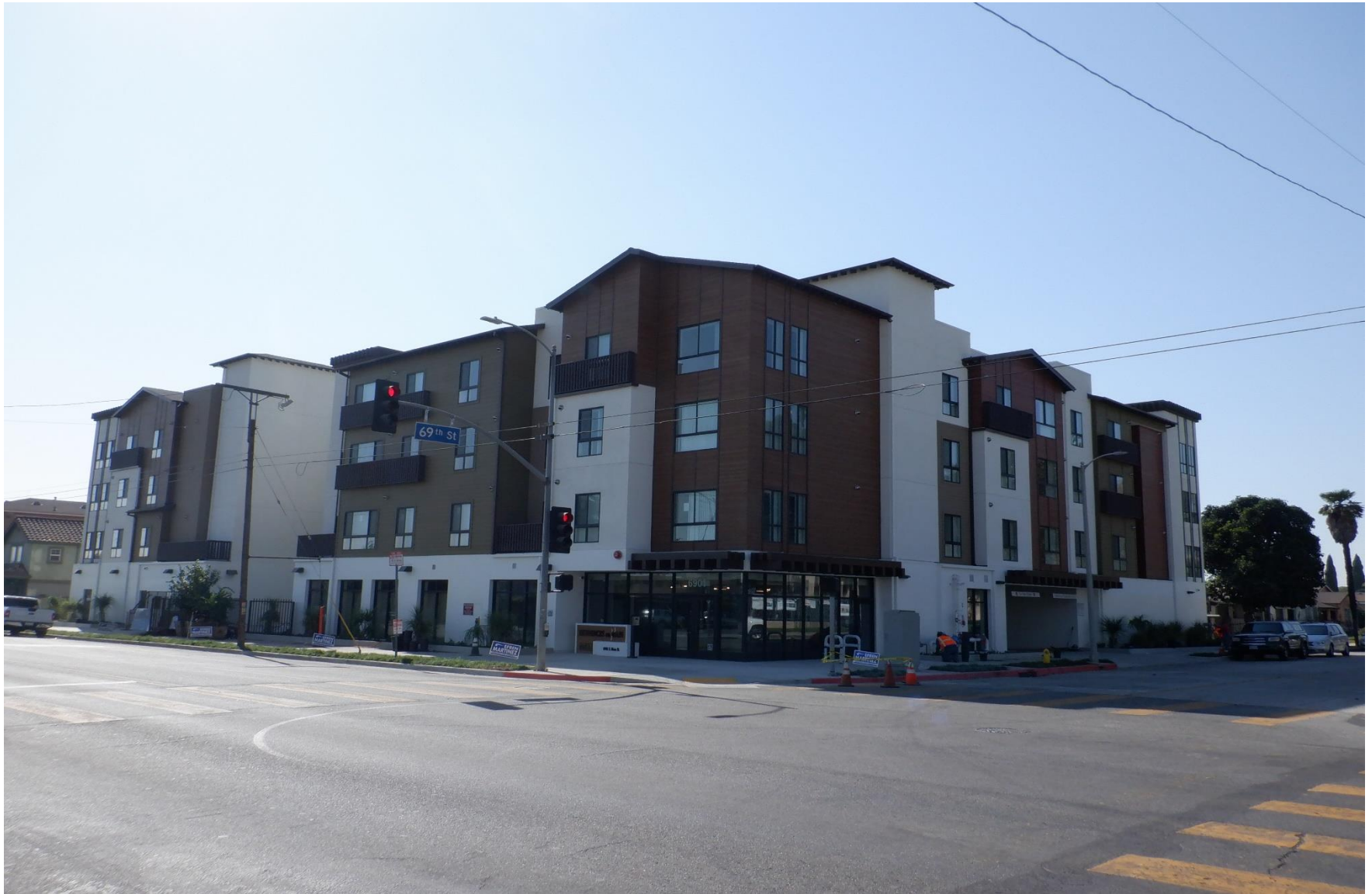
View from across the street on Main & 69 th St.
