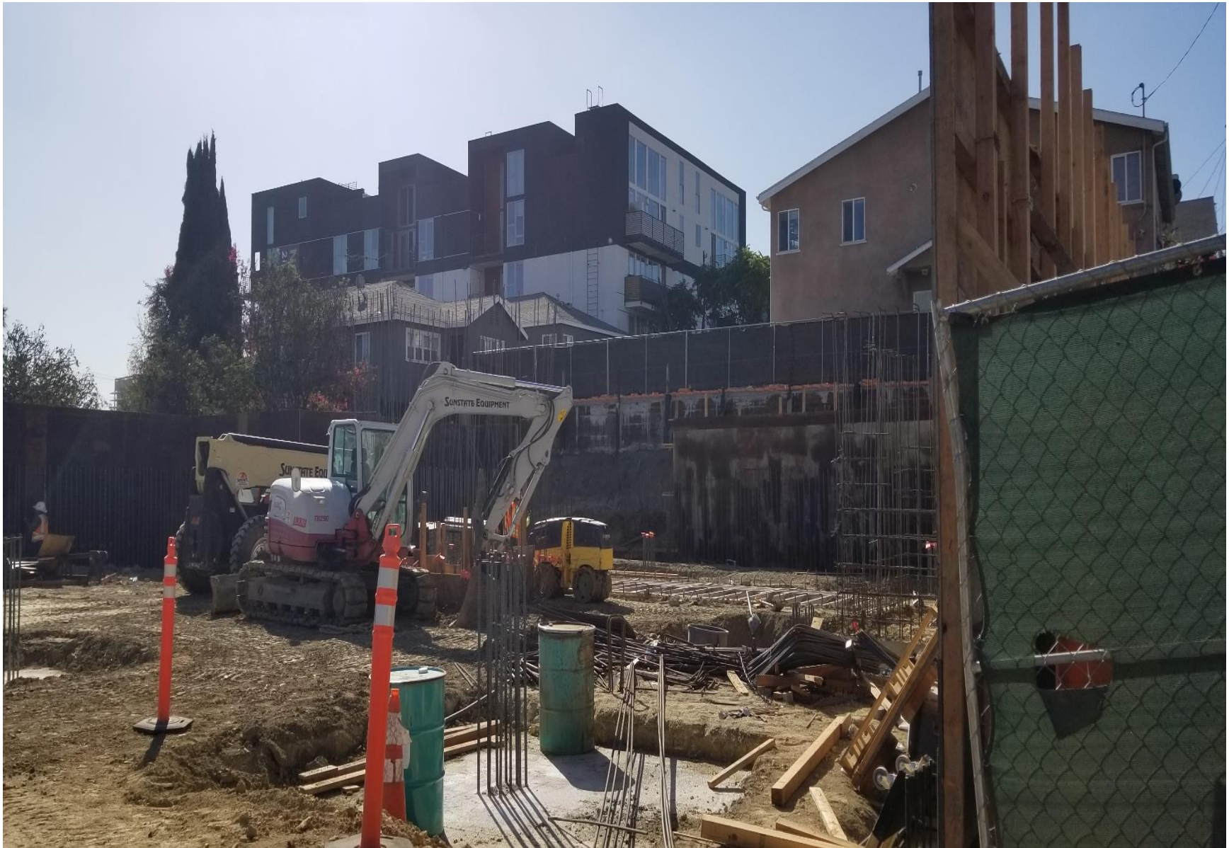
View from inside the fence at 418 Firmin St.
