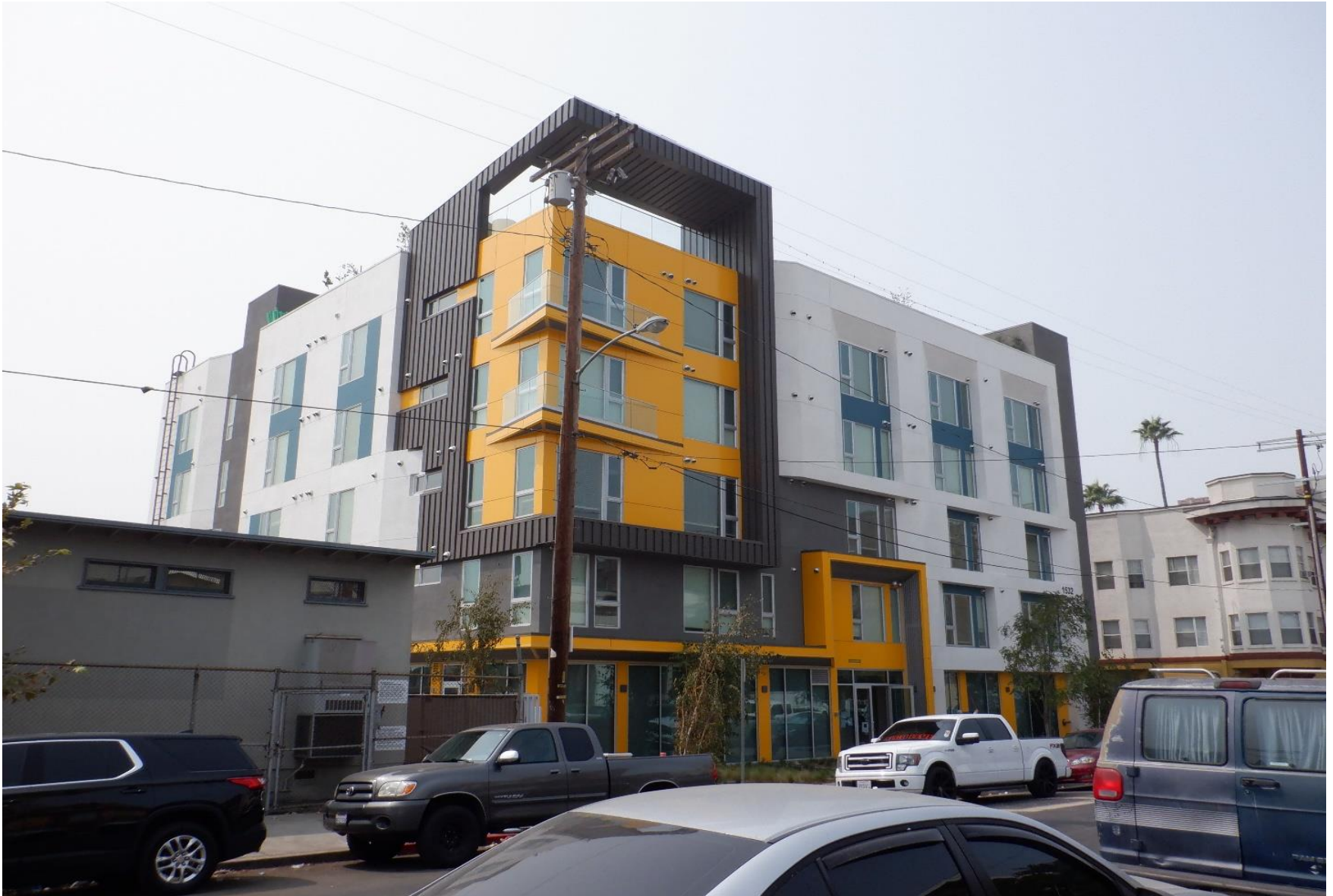
Located at 1532-38 Cambria St. View from across the street of site.
