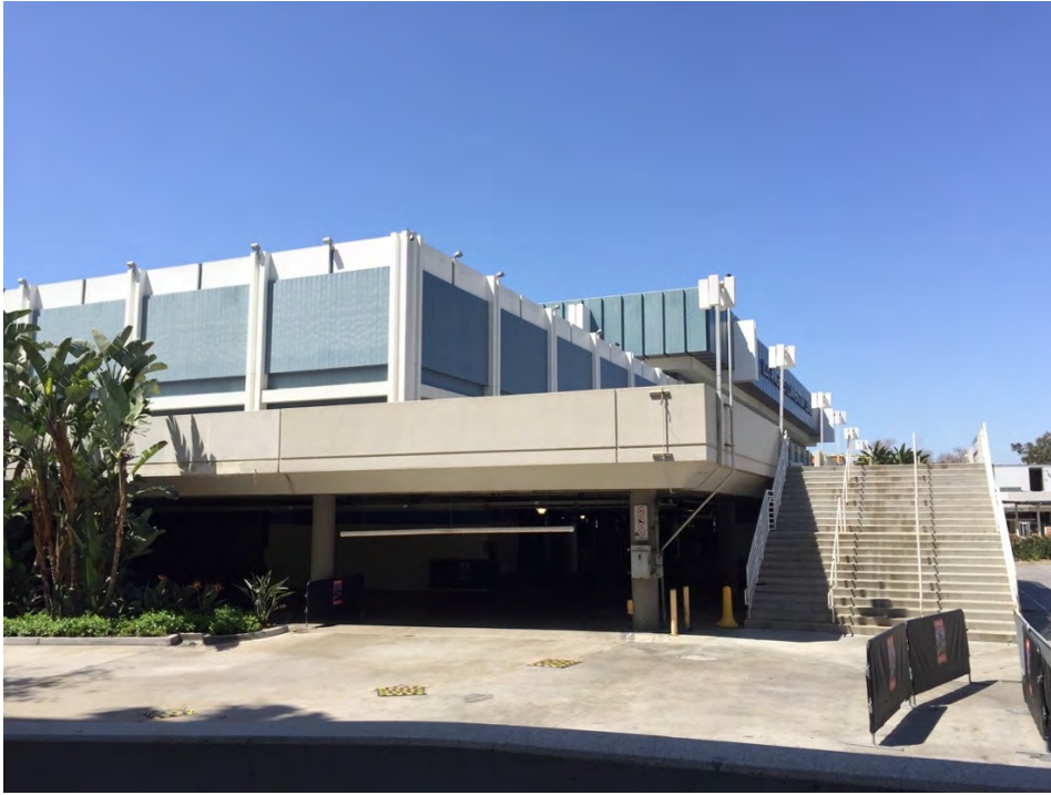
Figure 5: West Hall, showing the parking structure under, 'low-roof' and 'high-roof' structures
