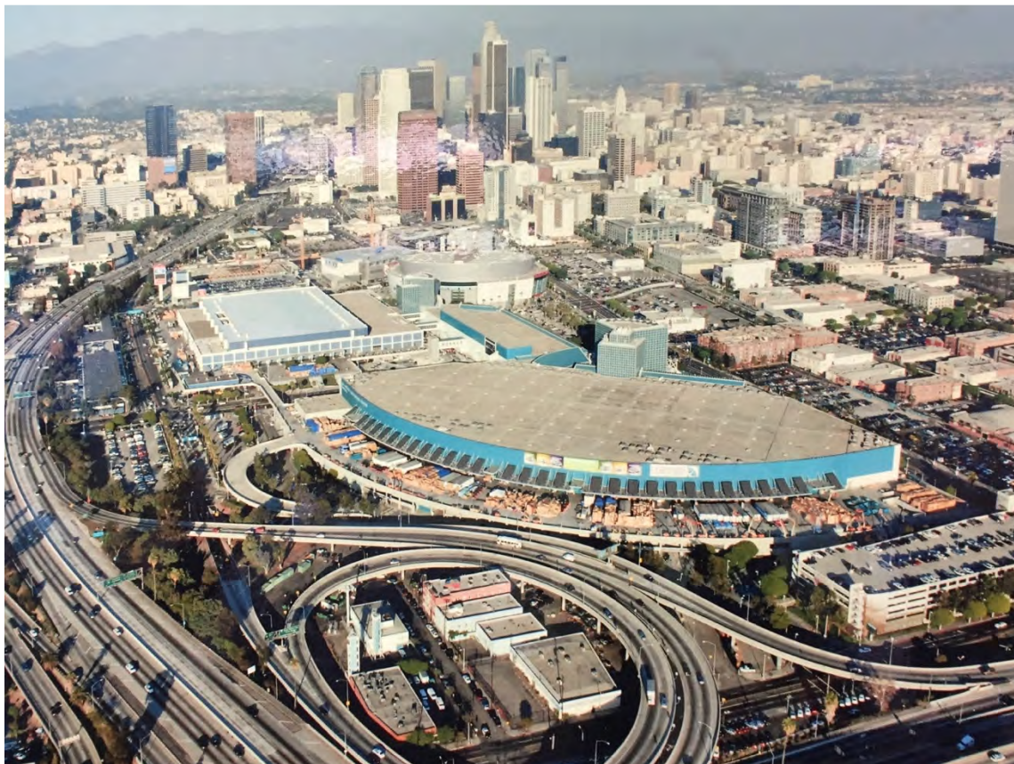
Figure 1: The LA Convention Center, with the West Hall in background, and the South Hall in the foreground.
