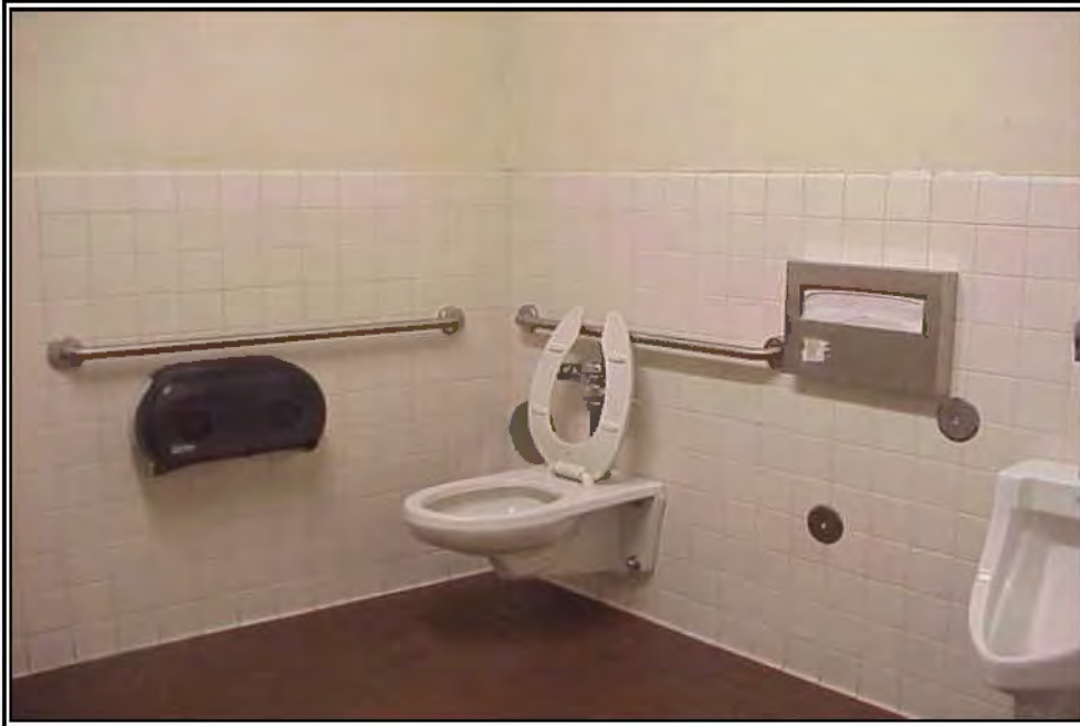
View of the men's restroom of the library/community center building
