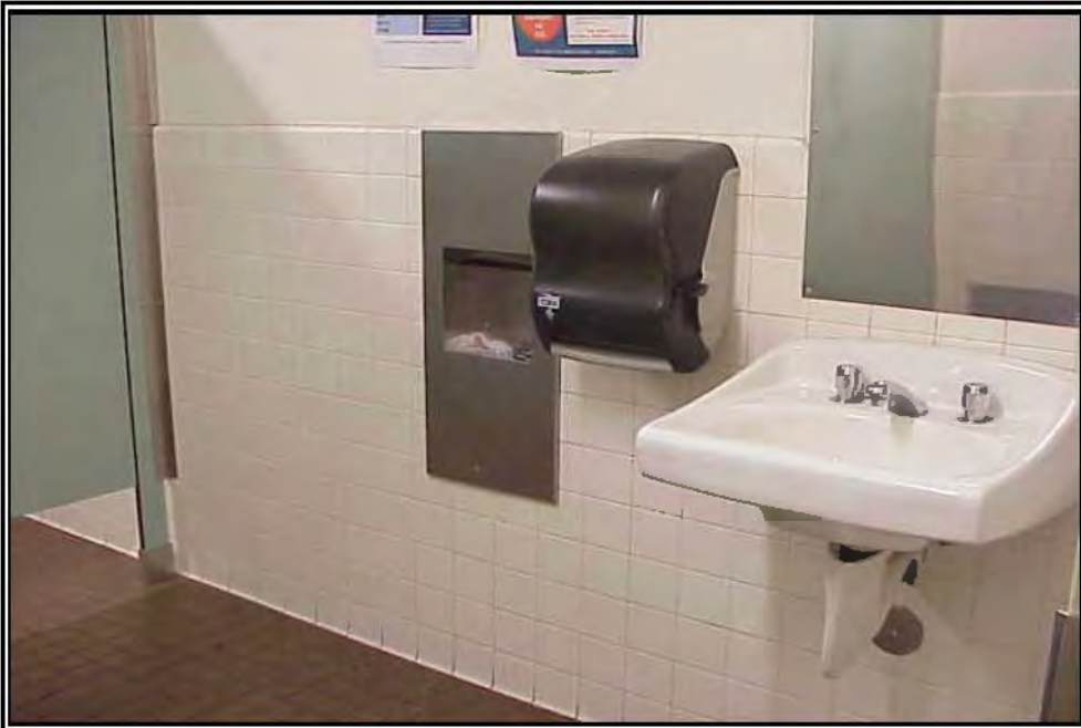
Partial view of the woman's restroom of the library/community center building
