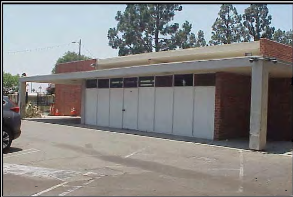
View of the east elevation of the subject property looking southwest from the on-site parking area
