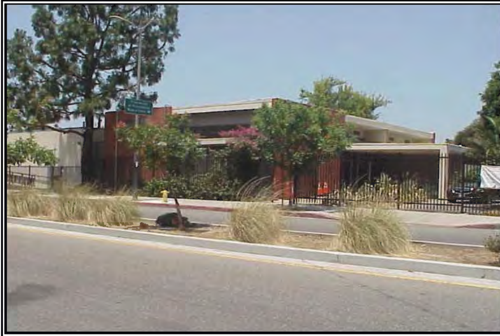
View of the south elevation of the subject property looking northwest from E. 103 rd Street
