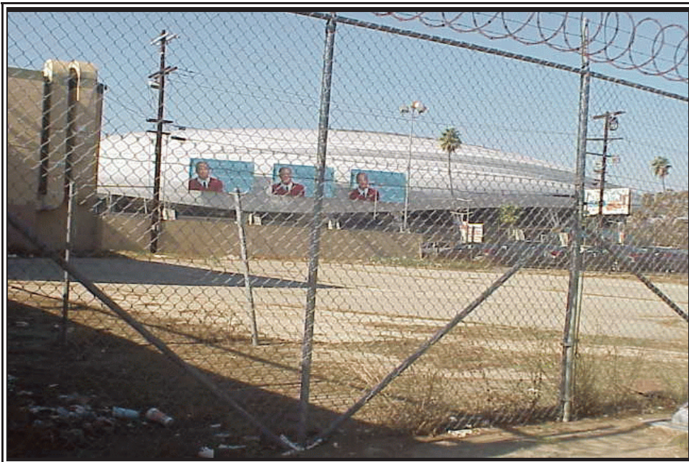
View looking northwest from the southeast corner
