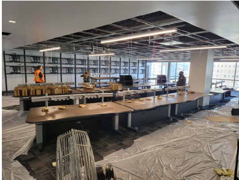
VIEW OF CONTROL ROOM
