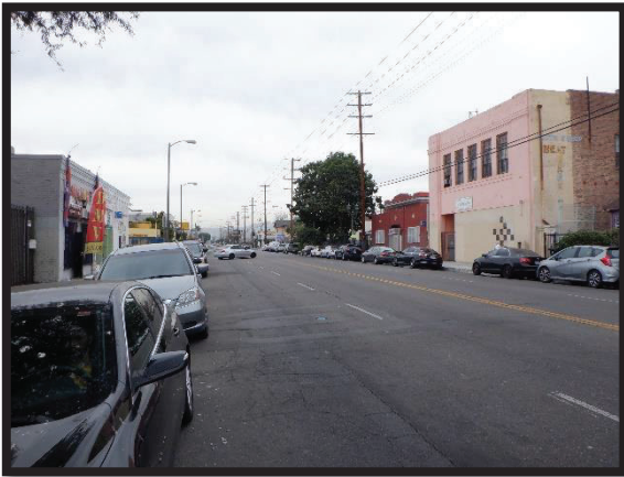
S. Main Street looking northerly
