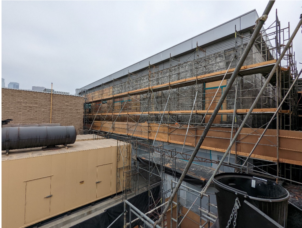
Erected scaffolding south side of FS4 facility
