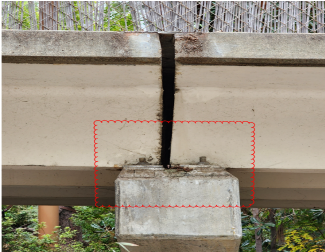
Offset Concrete Girder
