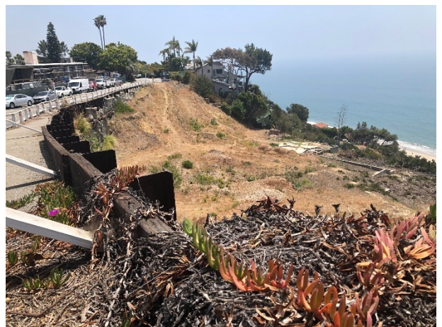
VIEW OF NORTHERN BORDER OF SUBJECT, LOOKING EAST
