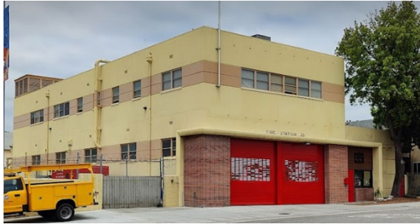
Fire Station #35 Apparatus Door Replacement
