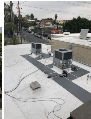
Fire Station #2 HVAC Replacement
