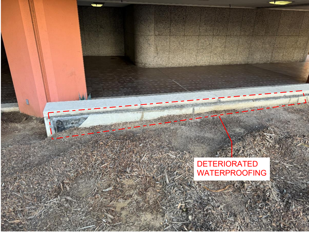
Photo 8: Deteriorated Waterproofing at Planter Walls
