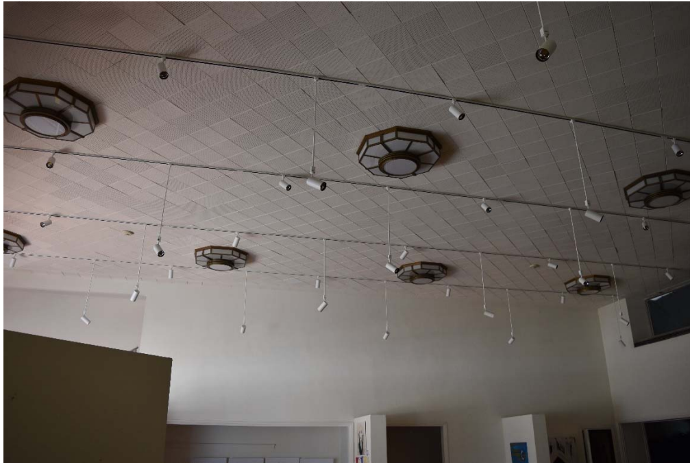
Phase I – LED Lighting Upgrade
