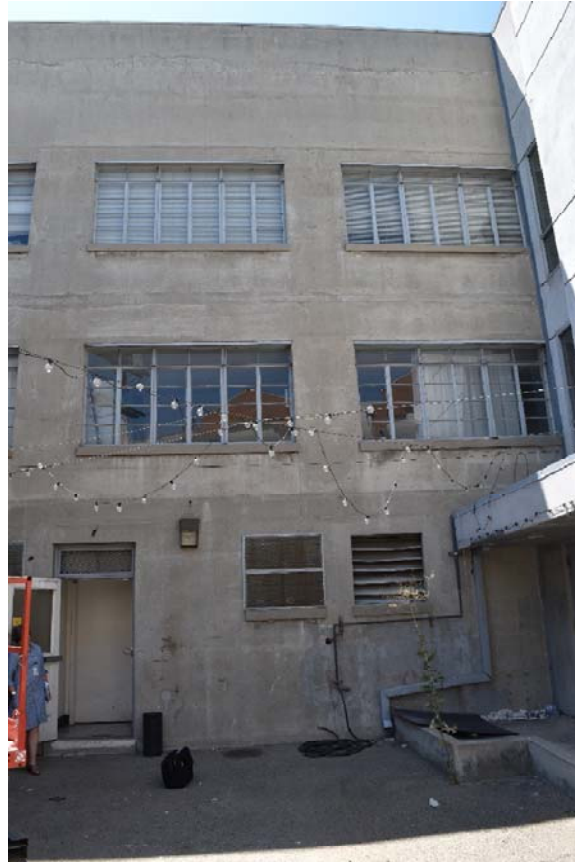
Phase II – East Wall Structural Sseismic Reinforcement Repair
