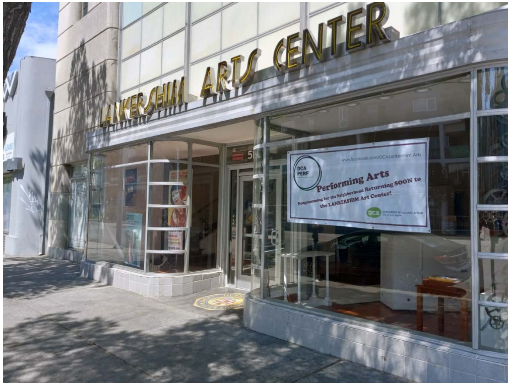
Phase I - Historic restoration of the storefront window
