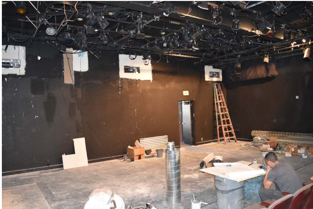
Phase I - Upgrades to Mechanical/HVAC components
