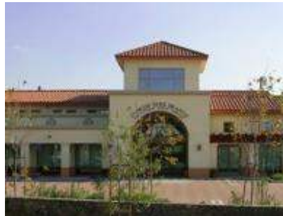
Cypress Branch Library Electrification, Efficiency, PV, BESS
