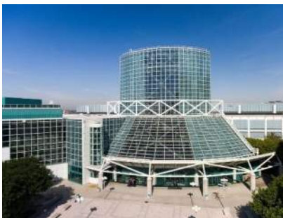
Convention Center Electrification, Efficiency, PV
