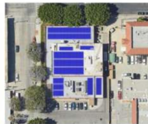
Hollywood Police Station
