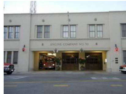
Old Fire Station #39 Electrification, Efficiency, PV, BESS
