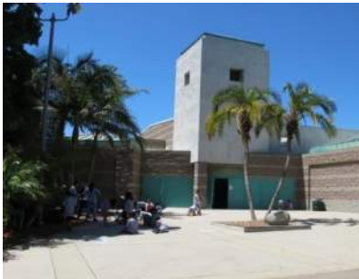
Balboa Sports Complex Electrification, PV, BESS
