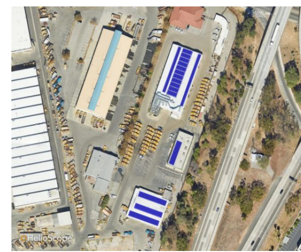
7th St Maintenance Facility (CD 14)
