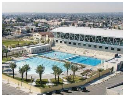
Expo Center Electrification, Efficiency
