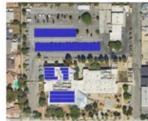
Topanga Police Station
