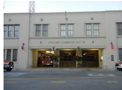
Old Fire Station #39 Electrification, Efficiency, PV, BESS
