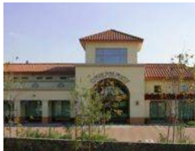
Cypress Park Branch Library Electrification, Efficiency, PV, BESS
