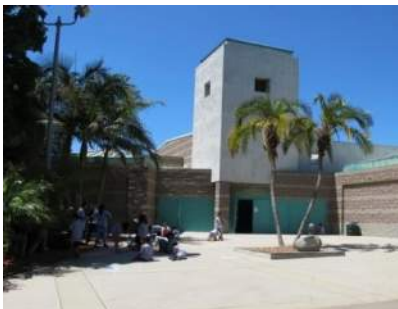
Balboa Sports Complex Electrification, PV, BESS
