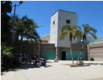
Balboa Sports Complex Electrification, PV, BESS
