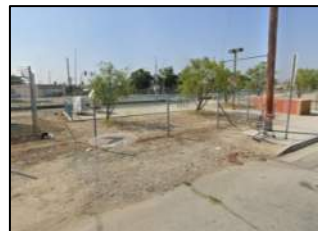
Photo: Metrolink station, view from San Fernando Rd.
