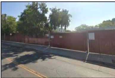
Photo: Existing condition of the school, view from N Normandie Ave.
