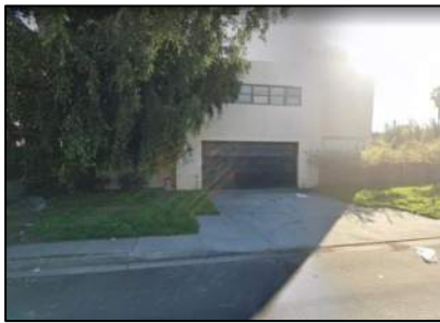
Photo: Existing condition of the former fire station, view from W 85 th Pl.
