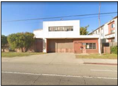
Photo: Existing condition of the former fire station, view from W Manchester Ave.
