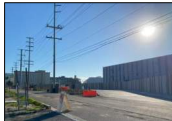
Photo: Existing condition of the site. View from the Cienega Blvd.
