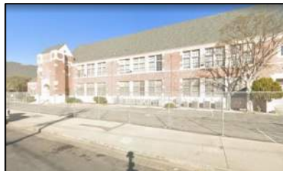
Photo: Existing condition of the school driveway from Gulf Ave.
