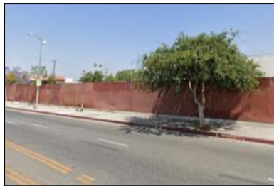
Photo: Existing condition of the school, view from Santa Monica Blvd.
