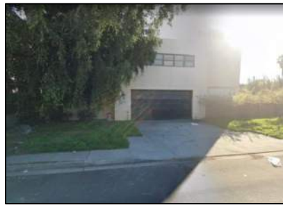
Photo: Existing condition of the former fire station, view from W 85 th Pl.
