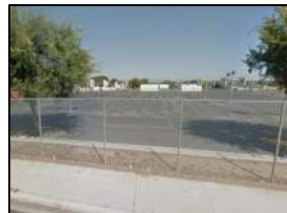
Photo: Existing condition of Beethoven Elementary School's paved playground, view from Lucille Ave.
