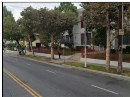
Photo: Existing condition of the school, view from S Wilton Pl.
