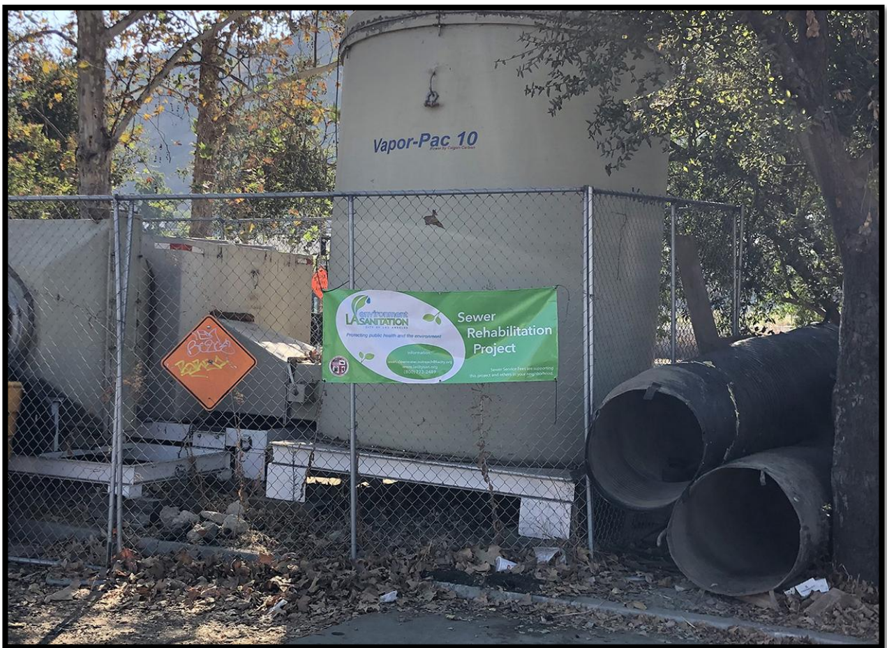
Figure B-1 – Construction Banner (Sewer Rehabilitation)
