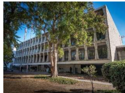
Van Nuys Police Station Electrification, Efficiency
