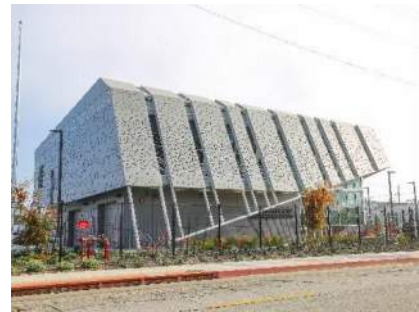
North Hollywood Sewer Yard
