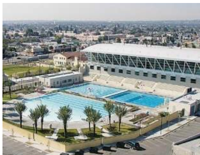
Expo Center Electrification, Efficiency
