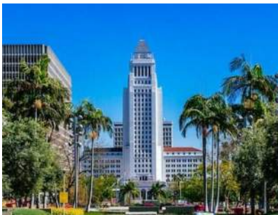
City Hall Electrification, Efficiency
