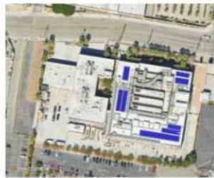
Emergency Operations Center
