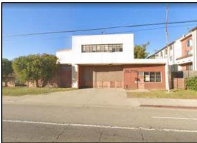
Photo: Existing condition of the former fire station, view from W Manchester Ave.
