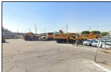
Photo: Existing condition of the City yard: proposed infiltration gallery area.
