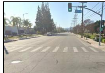
Photo: Plummer St facing west from Mason St.
