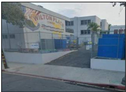
Photo: Existing condition of the school, view from W 8 th St.
