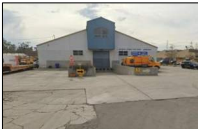
Photo: Existing condition of the City yard: front gate area.
