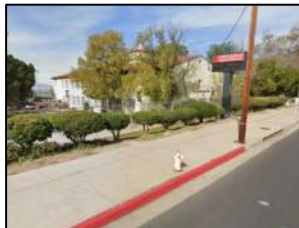
Photo: Existing condition of the school, view from Plainview Ave.
