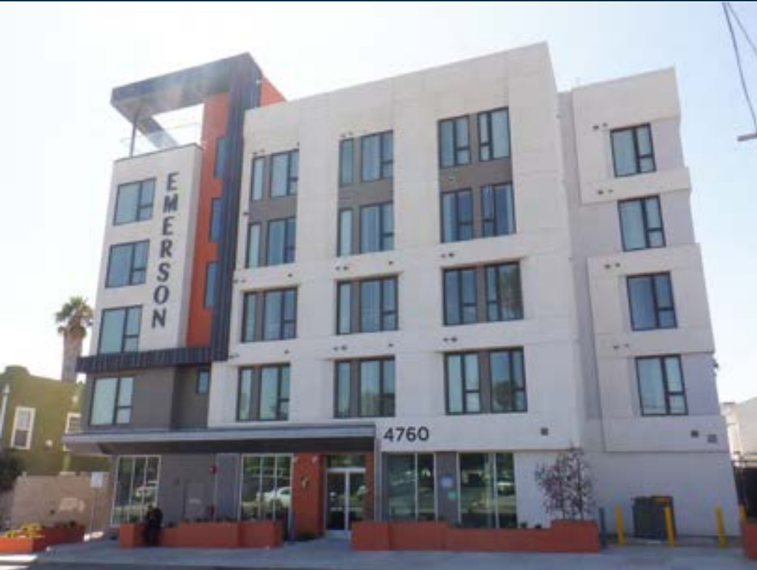
View from across the street at 4760 Melrose Ave.
