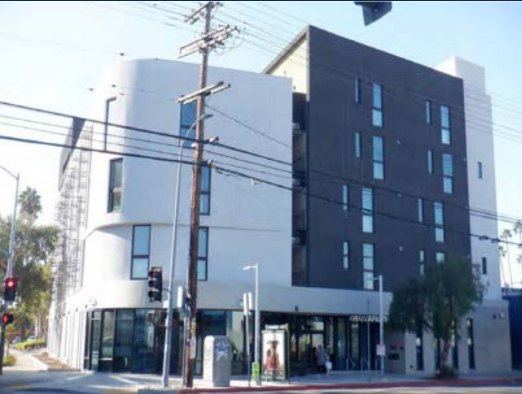
View from across Pico Blvd located on 4200 W Pico Blvd
