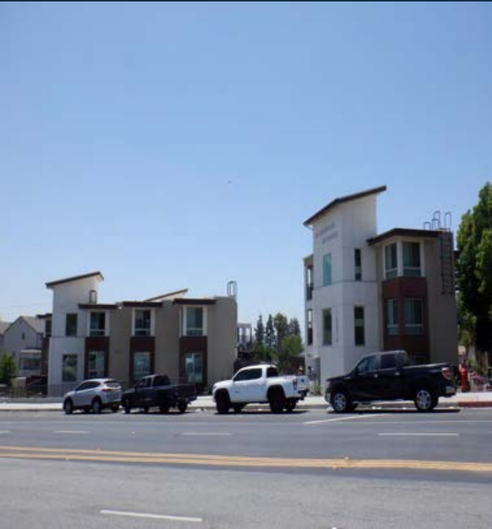
View of the buildings from the front of the site at 13574 Foothill Blvd.
